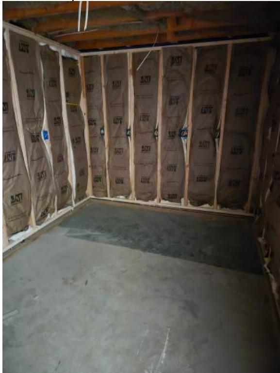
Room composition under construction
